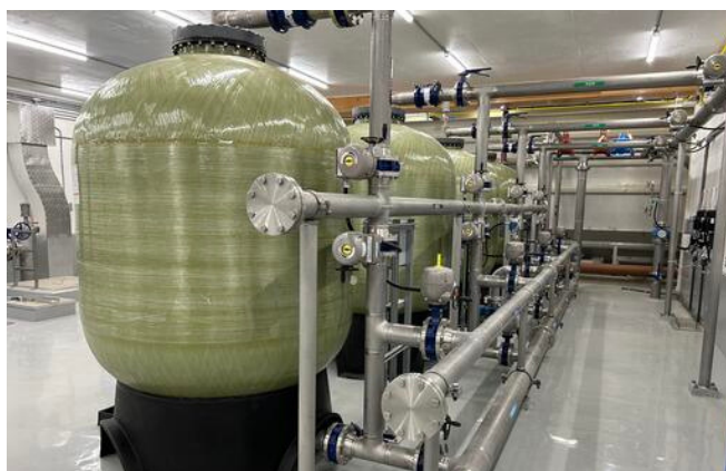
Arthur AYM Water Treatment Plant
